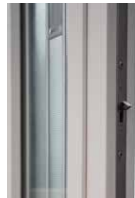
Multi-Point Locking System on Venting Sidelite
